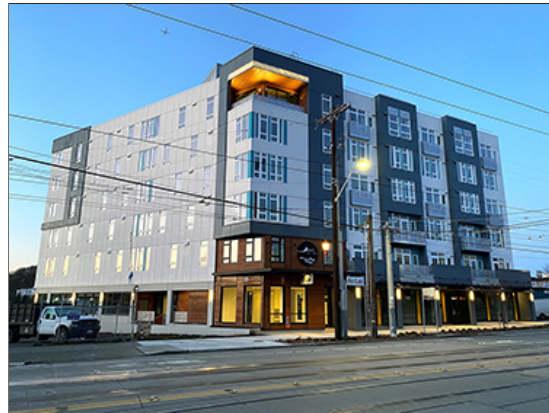
Exterior photo from Walsh Construction Co. [enlarge]
